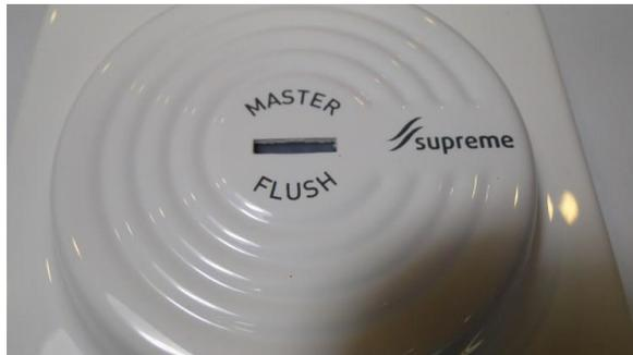
**Slot in sensor housing to be parallel to the urinal, not at right angles.**
