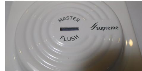
Slot in sensor housing to be parallel to the urinal, not at right angles.
